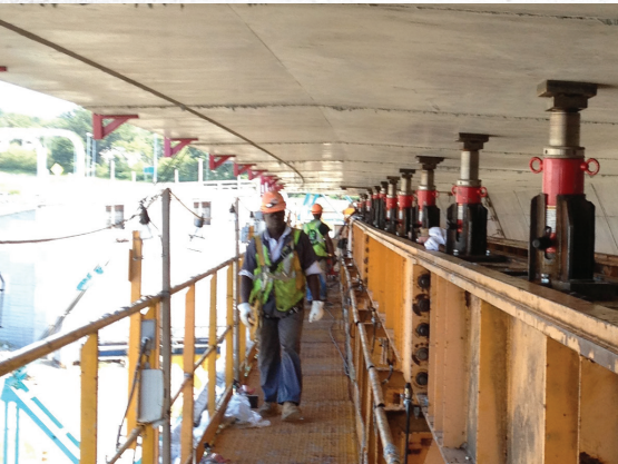
(42) HLN5508 cylinders lifting the Jordan Bridge in Cheasapeake, VA.
